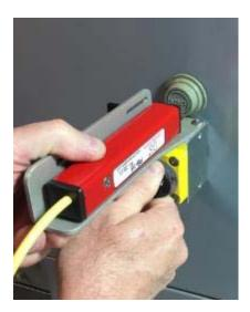
**STEP 4** – At this point the actuator should be firmly attached to the switchgear door with the plunger tip over your button.
