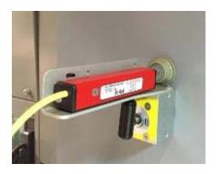
The magnet should be firmly against the switchgear door. If the magnet is not set firmly against the door, it will likely not have enough holding power to stay on the door when actuated.
