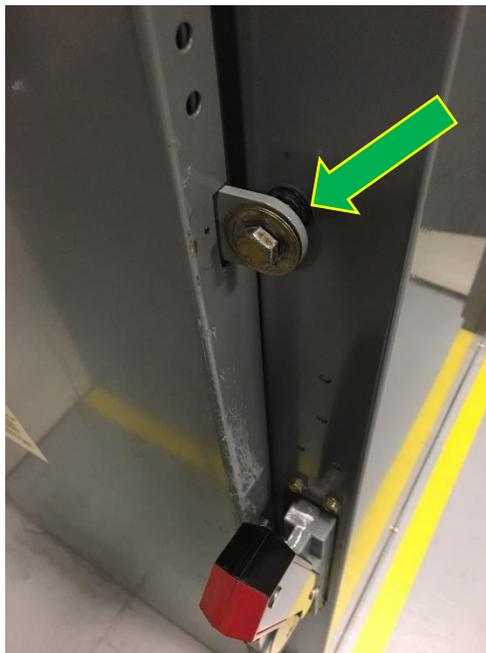
**STEP 2** – Prior to installing the ABL3 actuator, verify that the magnets are in the OFF position. Start with the ABL3 held low on the switch. Slip the actuator arm under the operating handle and move the up and over the operating handle mechanism.
