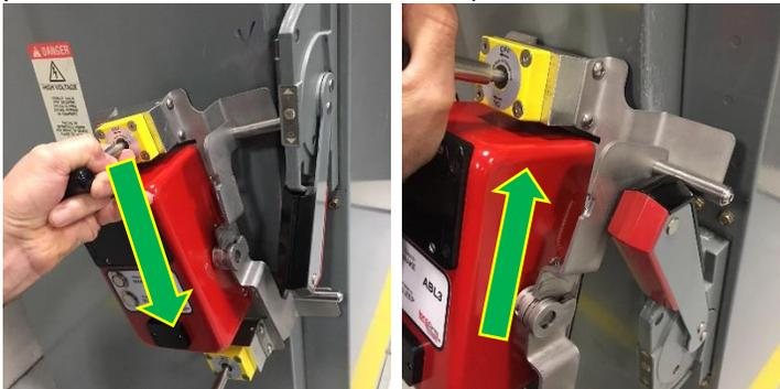
**STEP 4** -- Disconnect cable (for cabled versions only) and return components to carrying case or store on the side of the MCC. (See Section 5.0 for details)
