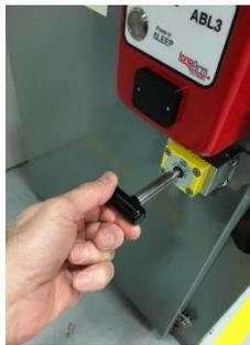
**STEP 3** – Raise or lower the actuator off the operating handle (depending on the position of the disconnect handle).
